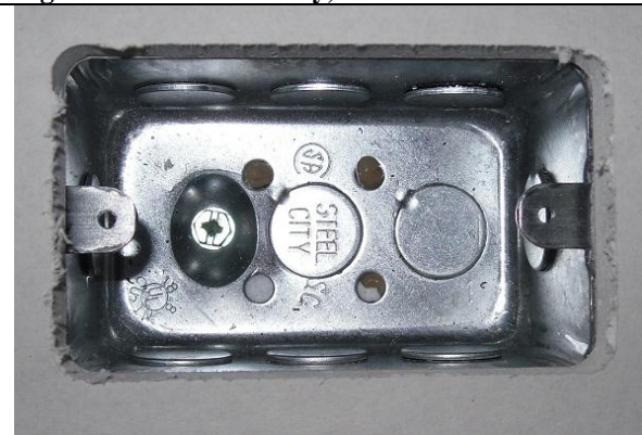
Figure 5 - Outlet box, installed in panel
