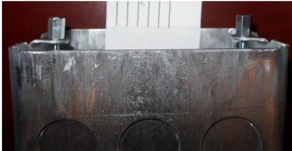
Photo 9 - Outlet box, with extension screws side view
