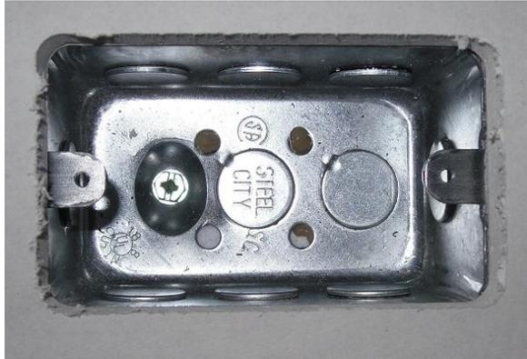
Photo 7 - Outlet box, installed in panel
