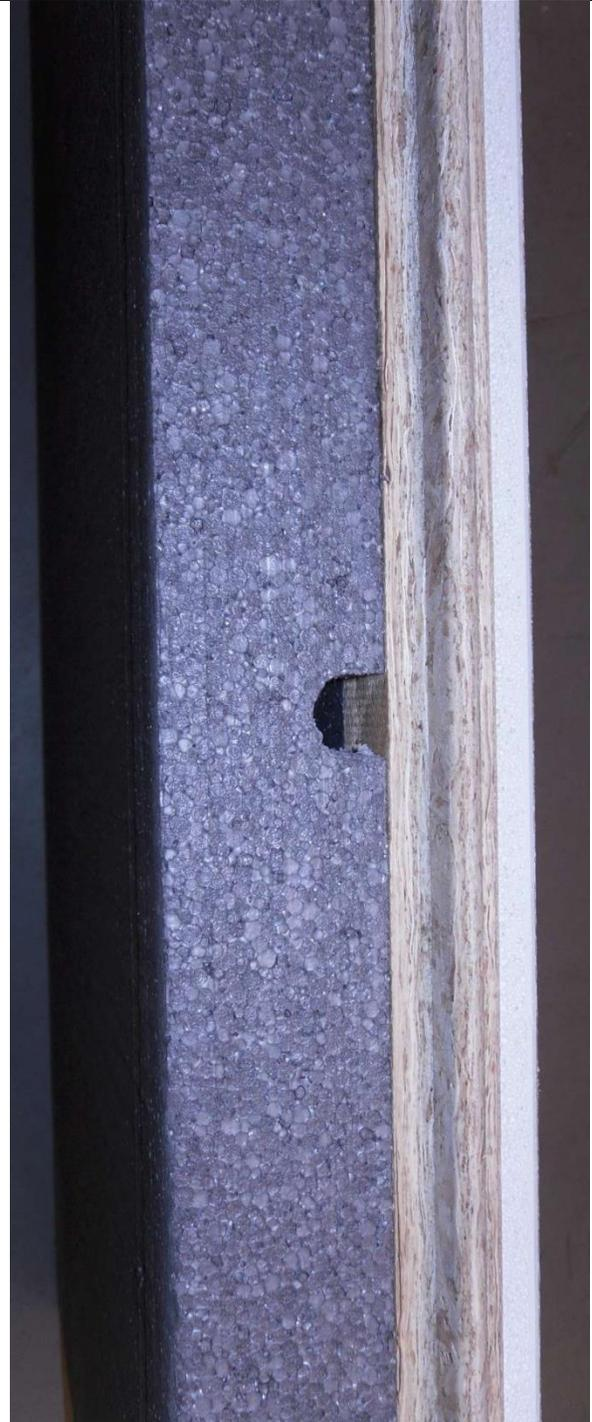
**Photo 2 - Wall Assembly, Side View**
