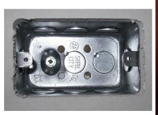
Photo 7 - Outlet box, installed in panel
