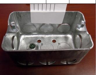
Photo 8 - Outlet box, with extension screws
