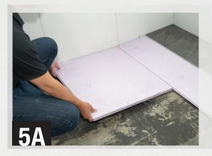
Work your way across the room installing one row at a time of the DRICORE Insul-Armor panels, then the finished floor treatment, until the room is complete. Remember to stagger the joints of the DRICORE Insul-Armor panels sufficiently row to row. Also, always follow the installation instructions of the finished floor as recommended by the manufacturer. Pay attention to acclimation requirements, and spacing at the room perimeter for expansion.
