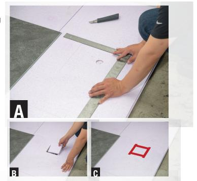
To protect your wall framing from moisture coming through the concrete slap, it is recommended to install DRICORE Insul-Armor directly beneath your framing. Cut strips of DRICORE Insul-Armor 3 1/2" wide, and install these strips beneath your wall framing. Remember to allow an additional 1" of space for DRICORE Insul-Armor panels when building walls. DRICORE Insul-Armor should be installed at the same time as the installation of the finished floor.
