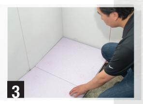
Install the first row of panels until you reach the end of that row, trimming the last panel to fit. If the resulting cut-off is greater than 18" long, you can use it to start the next run of panels. Make sure you install shims between the DRICORE Insul-Armor panels and the finished walls, so panels don't shift during installation.. Some installers prefer taping the joints of the panels with a vapor barrier rated tape to help hold the panels in the first 1-2 rows together during installation.
