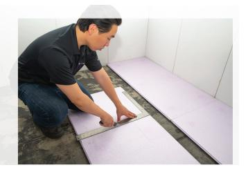
In the event that damage does happen to the DRICORE Insul-Armor panels after being installed, simply cut out the damaged area, replace with a fitted piece matching the cutout dimensions, and tape the seams using a vapor barrier rated tape (available at building supply stores in the vapor barrier section).
