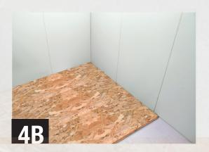
Install one of the recommended underlayment substrates below directly on top of DRICORE Insul-Armor.
