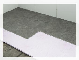
For optimal installation, it is recommended to use a self-levelling compound when installing over uneven floors. The maximum unsupported space beneath a DRICORE Insul-Armor dimple should not exceed the following based on your finished flooring type:
