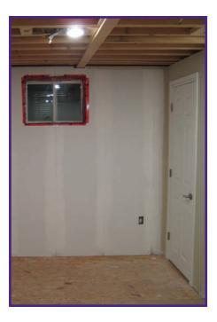
Cut the plywood into strips 4" wide and the height required for the door opening. Simply run a "squiggly" bead of P.L. Premium adhesive on the back of the plywood strips, and wedge them securely into place using scraps of lumber cut ½" wider than the opening between the plywood pieces once they are in place. Make sure the 5/8" rough frame strips are flush to the surface of the drywall. Let this glue set up for a minimum of 12 hours before removing the bracing and installing the door.
